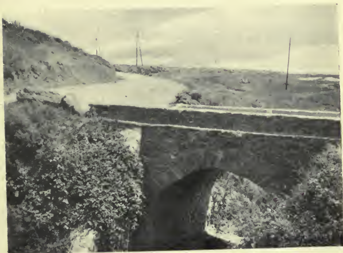
A BEND IN THE PASS WHERE SEVERAL ACCIDENTS OCCURRED BEFORE THE PROPER BRIDGE AND PARAPET WERE BUILT
